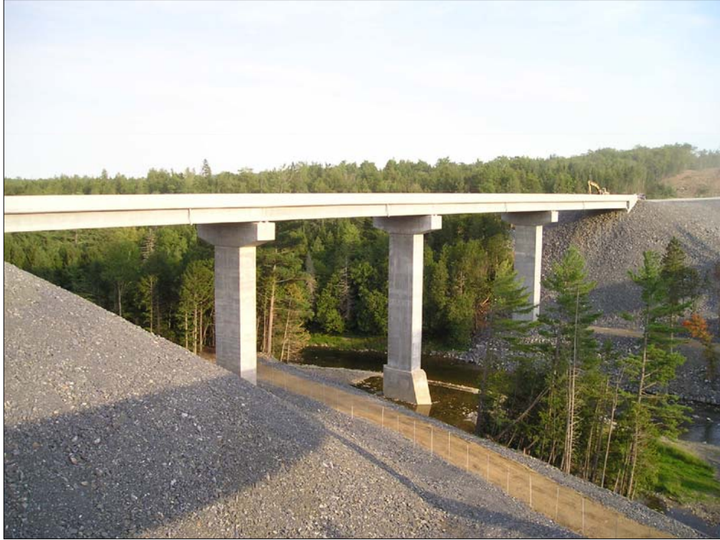
BIG PRESQUE ISLE STREAM TRANS-CANADA HIGHWAY PROJECT, NB
