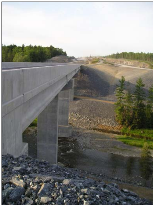
BIG PRESQUE ISLE STREAM TRANS-CANADA HIGHWAY PROJECT, NB
