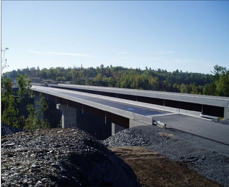
JEWETTS CREEK BRIDGE No. 2 LONGS CREEK, NB
