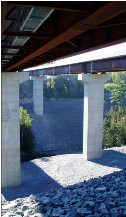
JEWETTS CREEK BRIDGE No. 2 LONGS CREEK, NB
