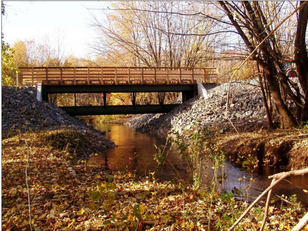
KILLARNEY BROOK TRAIL BRIDGE FREDERICTON, NB
